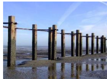
Close-up of a pile barrage
